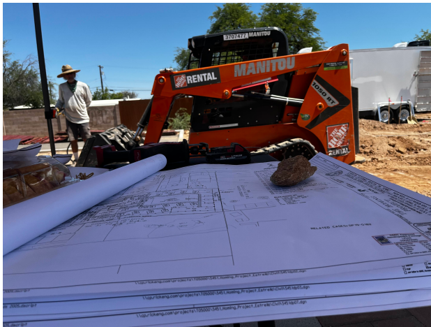
Left: Plans for the village guide the work. A machine for excavating the pathways is in the background.
